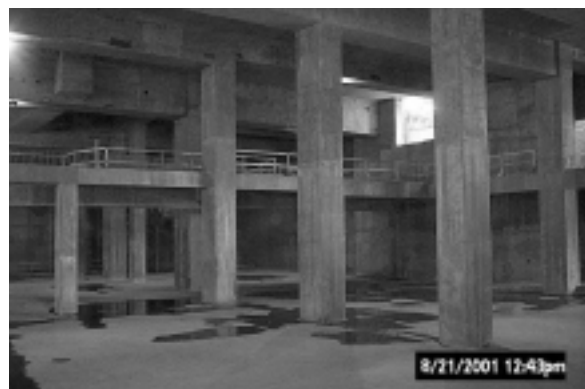
AFTERDISASTER® completed cleaning and decontamination
