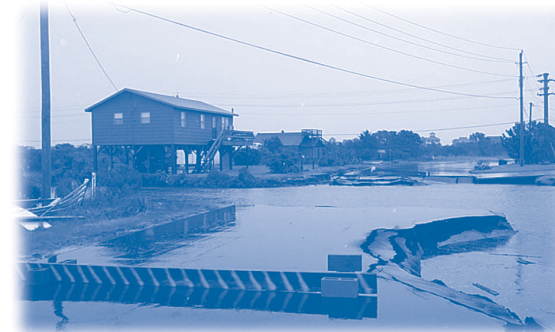
Hurricane Isabel washed away the highway connecting Hatteras Island to the mainland.
