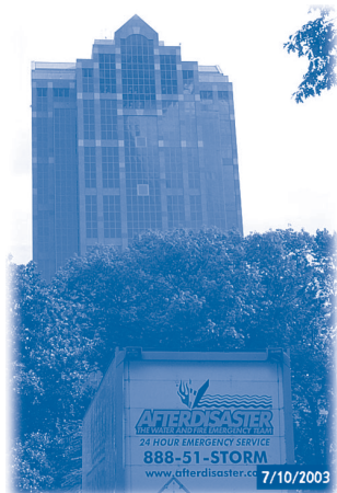
AFTERDISASTER has the expertise and equipment to mitigate damages and restore skyscrapers such as this one.
