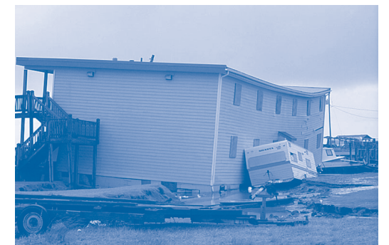
Sustained hurricane winds of 70+ mph and storm surges rearranged property.
