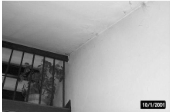
Soot tags result from smoke residue, even where there appears to be no soot. These were found on the ceiling on a second floor stairwell.
