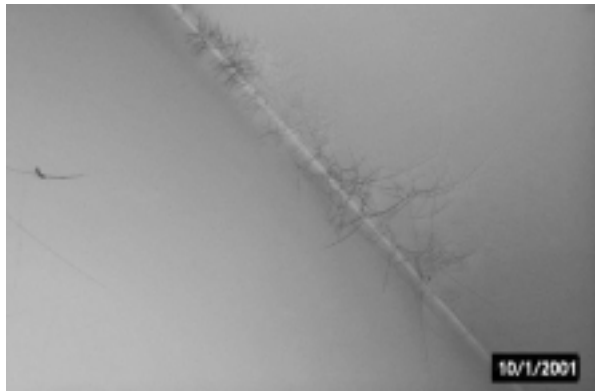
Soot tags result from smoke residue, even where there appears to be no soot. These were found on the ceiling on a second floor stairwell.
