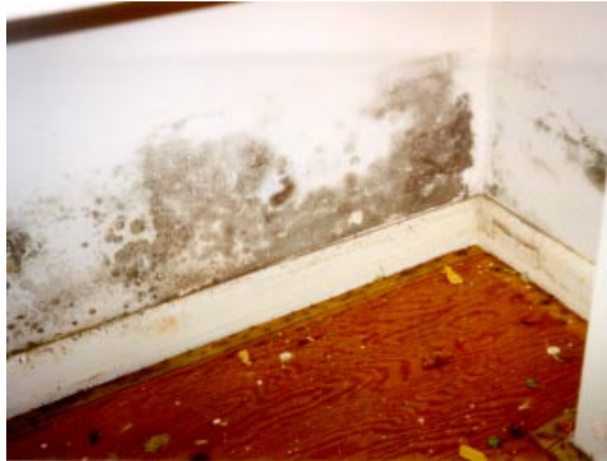
Aspergillus and Penicillium colonization on drywall
